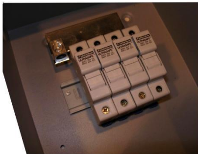
4 Touch safe fuseholders installed in an MNPV6
